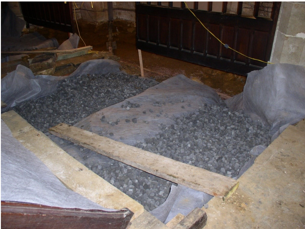
Fig. 4: Preservation measures below floor of new circulating area
