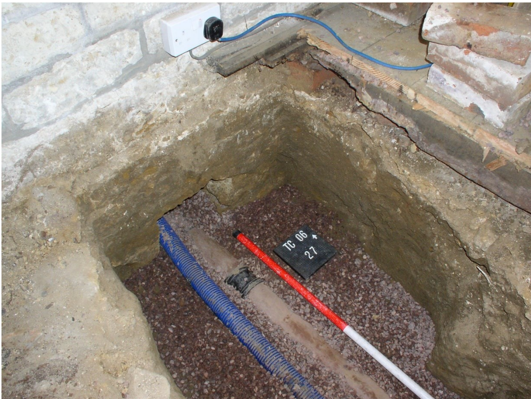
Fig. 14: Service trench, north aisle - foundation 27 (north wall) from south-west
