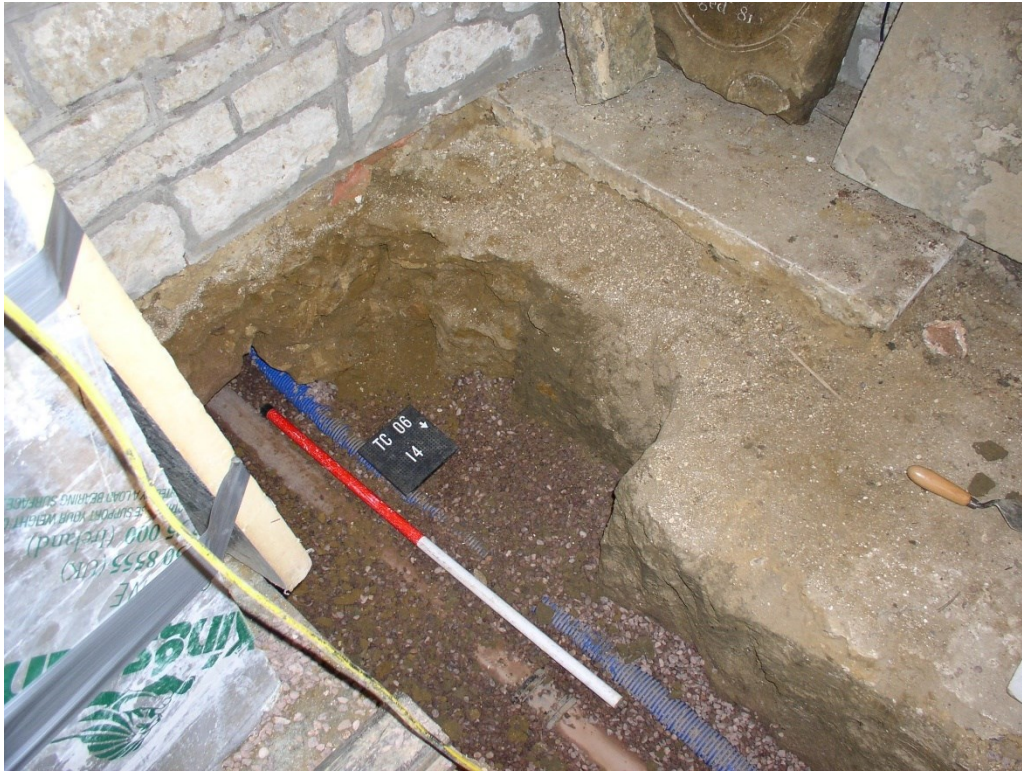
Fig. 13: Service trench, north aisle - foundation 14 (north arcade wall) from north-east
